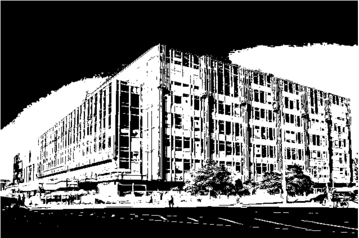
The Palast der Republik was built between 1973-1976 and was completely demolished to offer space for the reconstruction of the Stadtschloß in 2013
