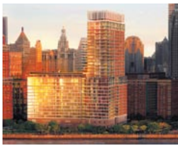
Riverhouse has solar panels and river views.
