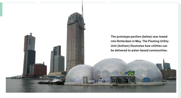
"Although we already have house-boats on the canals, this is the first floating structure in a harbor, which is subject to tidal conditions," Molenaar explains. Moreover, houseboats have hollow hulls that sink when they are punctured, while the pavilion has a lightweight foundation of expanded polystyrene reinforced with concrete beams, made buoyant by tiny air-permeated cells. "It is impossible to sink such a building," Roeffen says, "which makes it handy in getting a mortgage."
