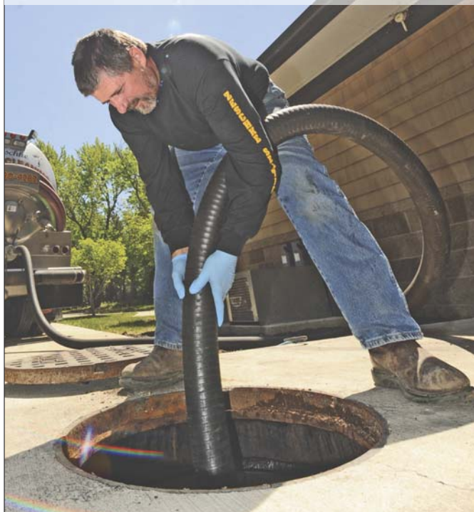
Cary Zeschke cleans a grease trap. Grease trap service has grown into about 30 percent of the company's business in eight years.
