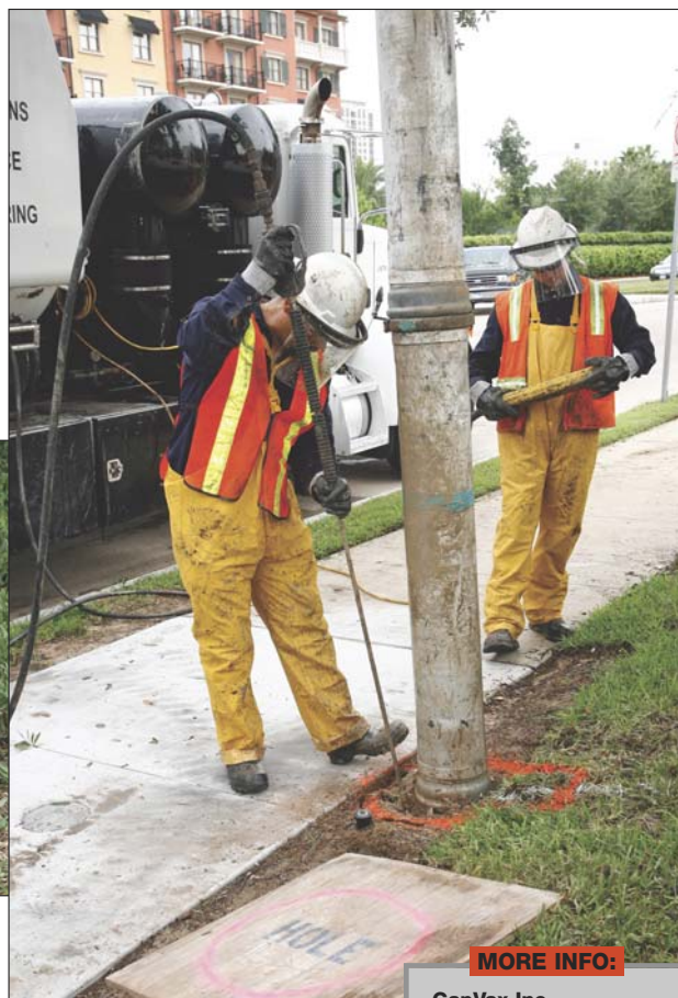
Water is jetted into each light pole hole, while mud is conveyed to the combination truck tank. At right, Rios and Pina monitor the hydroexcavation work.
