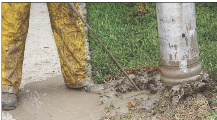
Water is jetted into each light pole hole, while mud is conveyed to the combination truck tank. At right, Rios and Pina monitor the hydroexcavation work.
