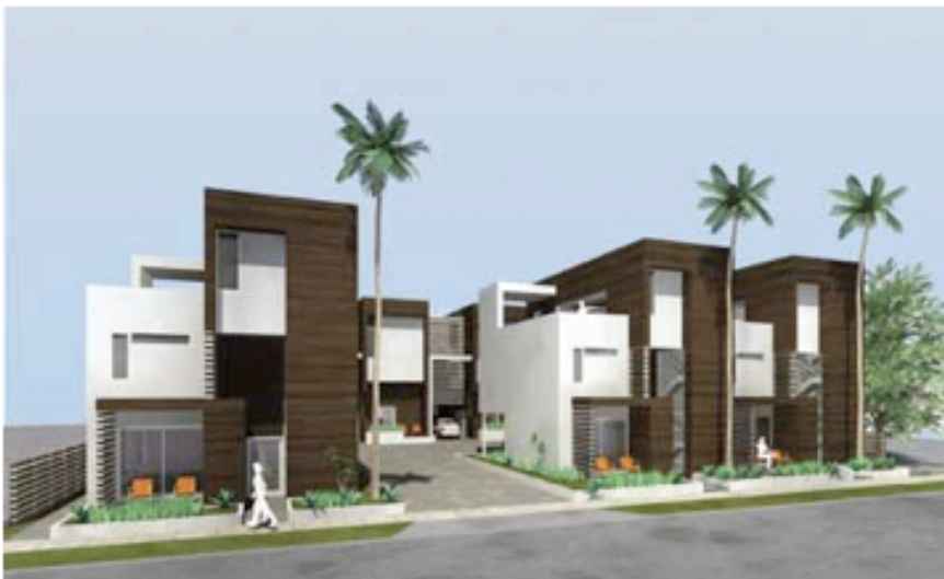
MODATIVE'S FAY AVENUE ARTS DISTRICT DWELLINGS, CULVER CITY.
