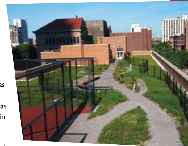
View of Ogden International School of Chicago's vegetative roof system from the building's northeast corner
