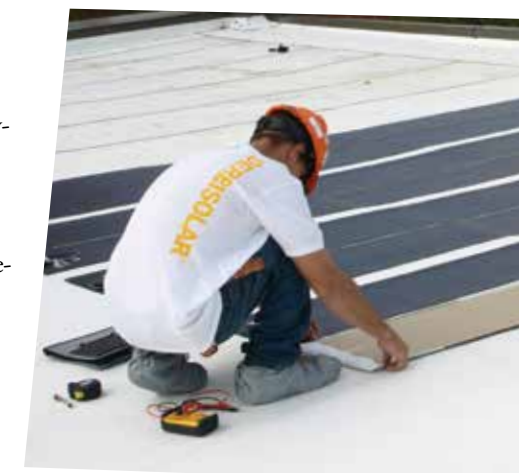
A Cornell Roofing & Sheet Metal employee installs solar panels on Bayer CropScience's roof system.
