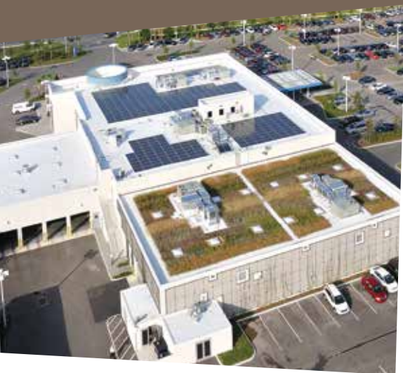
An aerial view of Headquarter Honda's roof system
